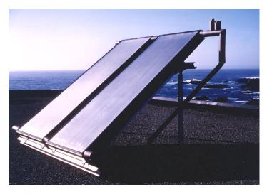
The collector(s) can be mounted on a South facing roof near the hot tub, or on a gazebo or even the ground, as long as they are higher than the hot tub or spa to allow draining back into the spa when not operating. If this is not feasible, a closed-loop heat exchange system should be installed.
