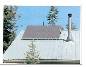
In retrofit situations, the perforated solar cladding can be applied over most existing walls and roofs. A few obstructions on a wall or roof should not present a problem.
