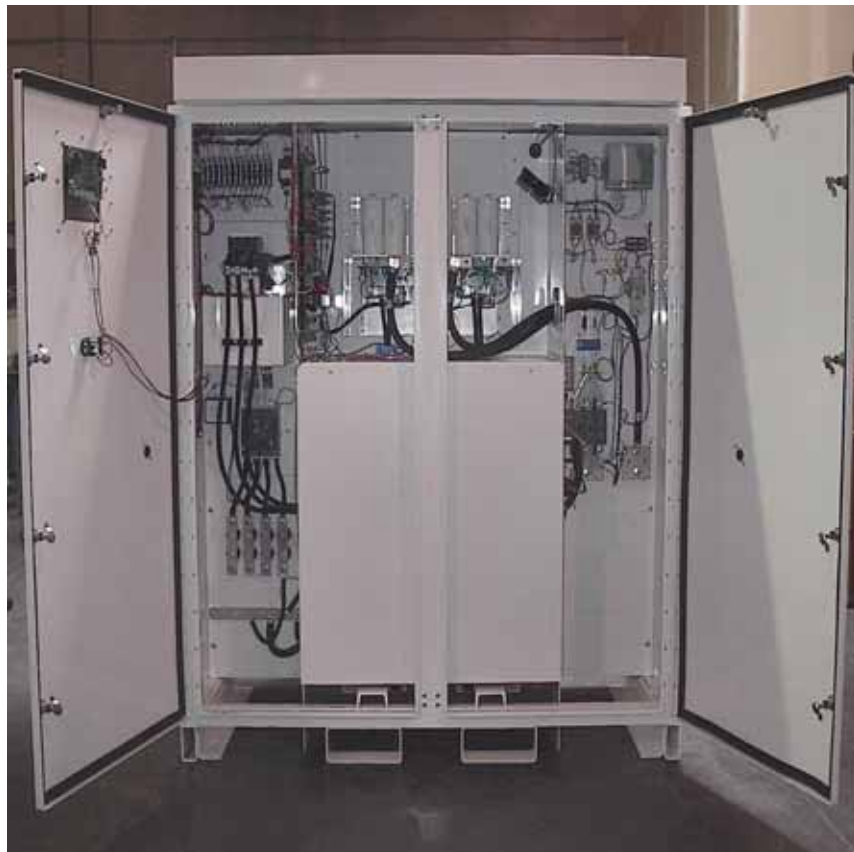
Figure 1-1 Main Inverter (Open Enclosure View)
